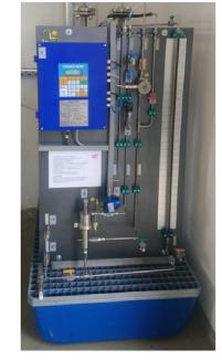
The core of our odorizing system type PD is WILLIAMS pneumatic dosing device. This device is self-sucking and do not require additional energy to suck odorant from the tank. The entire system of the odorization device is tight and made of materials that guarantee the reliability of the device and at the same time eliminate any leakage of the system.
