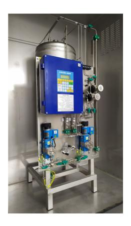
The odorization station is equipped with filters for capturing impurities in the odorant and also with a filter with activated carbon on the deaeration pipe. A level indicator is placed on the front panel in order to visibly monitor the amount of odorant in the tank, but also to verify the functionality of the dosing device.
