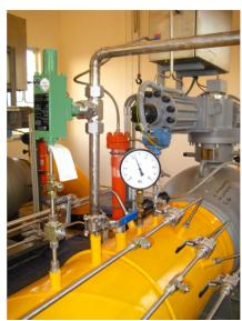
The basic requirement for the reconstruction of the GTS was the modernization of the entire equipment with remote control of the entire station from the regional control room without permanent operation of the GTS. GASCONTROL, s.r.o. , as the general contractor, was involved in the construction of a complex of interconnected equipment that allows unattended, remotely controlled, natural gas regulation to the HP gas network.
